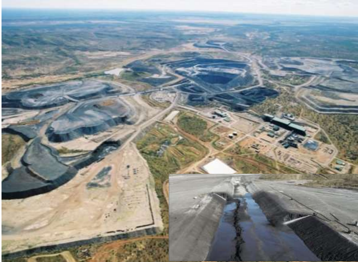
Century Mine, Queensland source: New Century Resources
